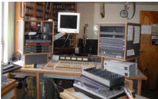
The old Control Room, being disassembled prior to rebuild.
